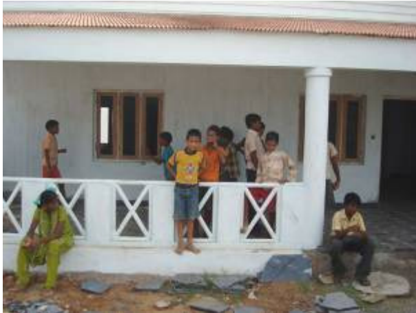
The construction of the Children's village is almost complete
