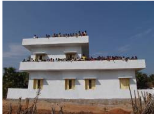
2 The second school, at Kotha Mukam:
